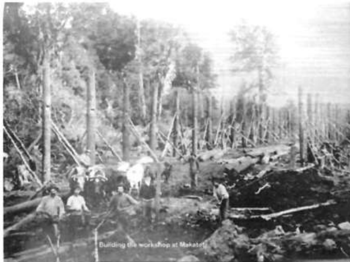
Building the workshop at Makatote, ca 1905.
