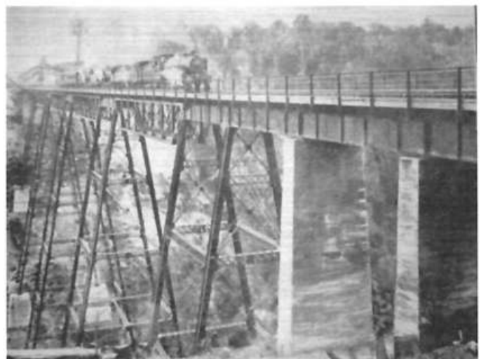
The test load train on the completed viaduct in 1908.
